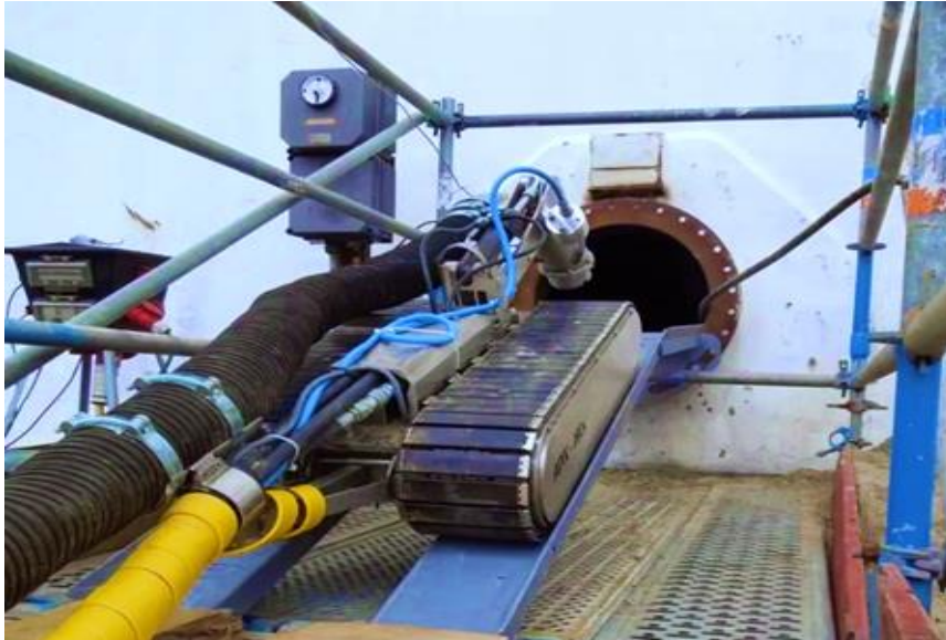
Fig. 6. Photo image - Cleaning process preparation
