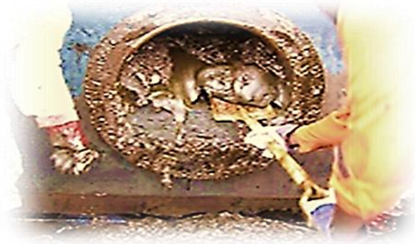
Fig. 3. Manual intervention - Oil sludge at the bottom of the crude oil tank [6],[8]
