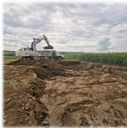
Photo 2. Excavation of polluted soil in the area of well 682 Suplacu de Barcău
