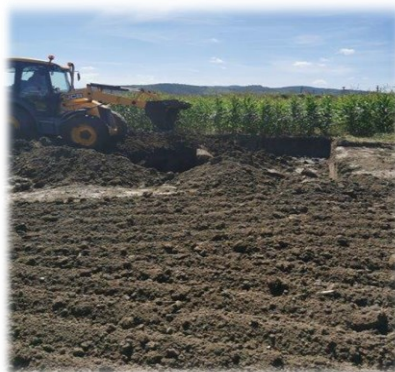
Photo 3. Replacement of polluted soil in the area of well 682 Suplacu de Barcău
