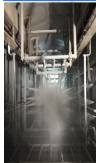
Car body washing with high-pressure spray nozzles to remove possible impurities
