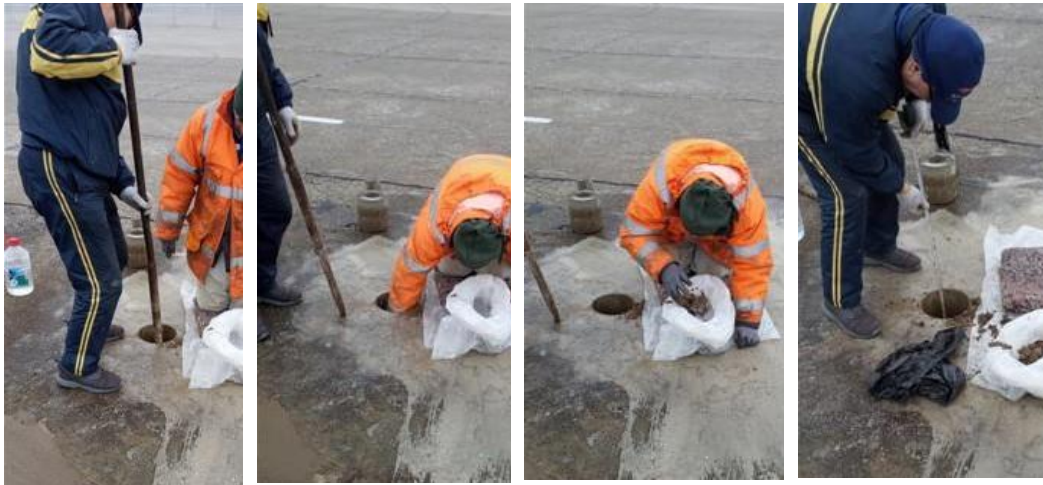
Fig. 4. Loosening the ballast with the crowbar, removing the ballast to ground level and measuring the thickness of the foundation layer
