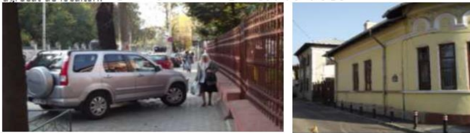
Fig. 3. Infrastructure for pedestrians occupied by vehicles parked illegally (left) and inaccessible to persons with reduced mobility (right)
