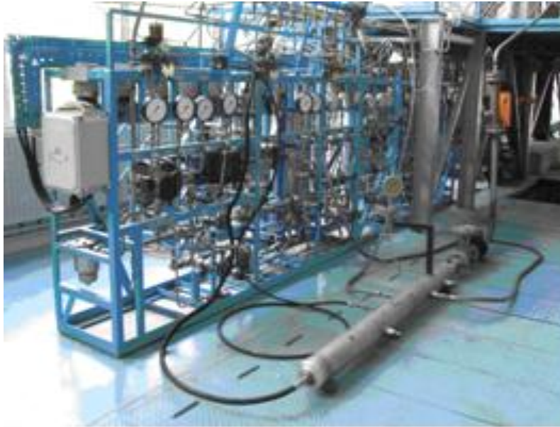
Fig. 9. The Mechanical Simulator installed at the valve station
