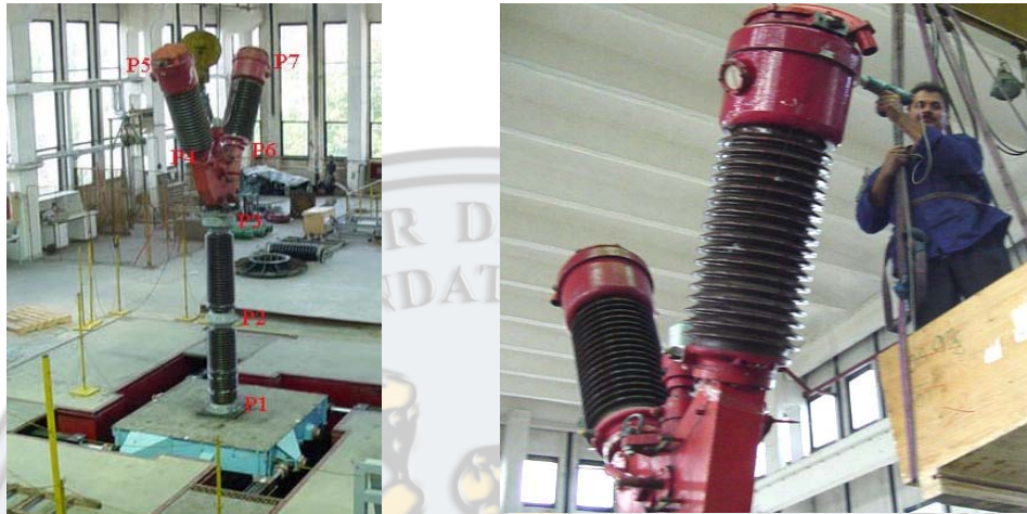
Fig. 1. Position of measurement and excitation points for IO 220 kV/2500A circuit breaker.
