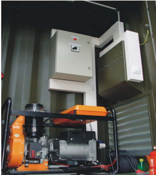
Fig.6. Inside view of the technical compartment with the back-up generator of the “C 4 I”
