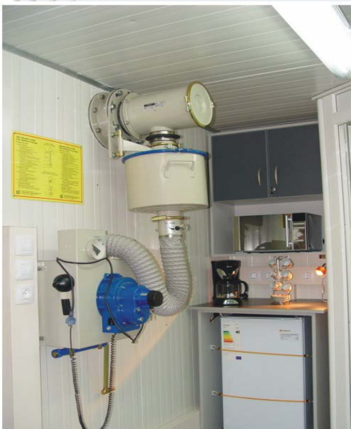
Fig. 8. Kitchen facility and NBC filtering system.
