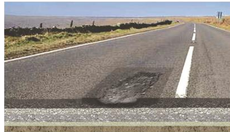
Fig. 12. Warming the defective area
