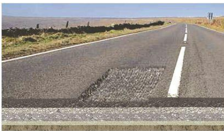
Fig. 11. Milling the defective area
