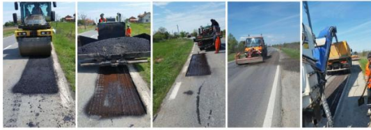
Fig. 9. Equipment required for classical technology.
