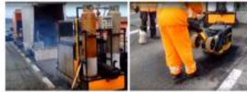
Fig. 10. Equipment needed for IR technology.
