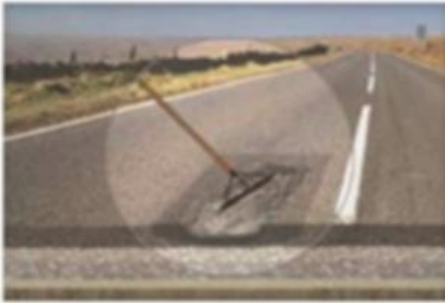
Fig. 3. Scarifying the heated zone
