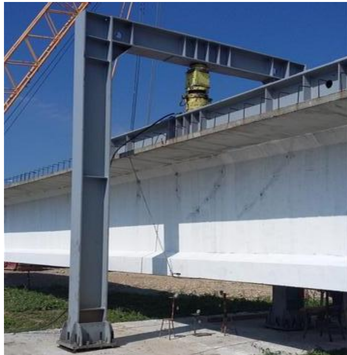
Fig. 1. Detailed frame location, press, intermediate metal beam, tensometric marks, comparators.
