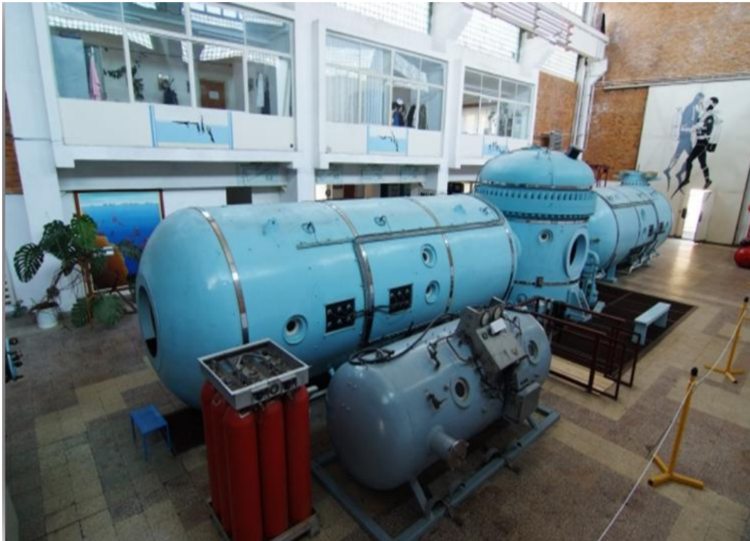
Fig. 1. - The Hyperbaric Complex of the Diving Center seen from behind.
