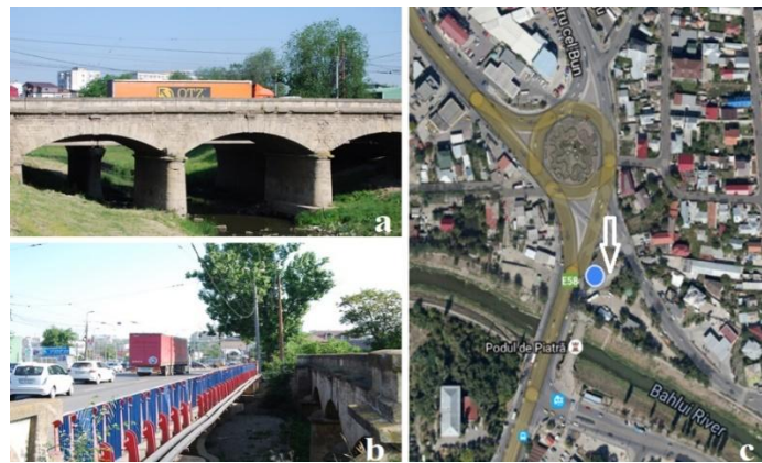
Fig. 2. Stone Bridge ( Podul de Piatra ) road junction Iasi, Romania. a - historical bridge; b – newer bridge; c –location of exposure area. [8]
