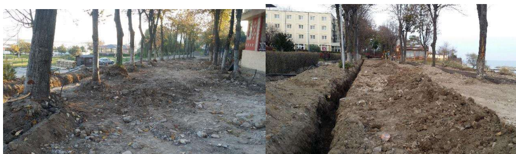
Fig. 7, 8 – Rehabilitation works of the Linden Alley in Mangalia
