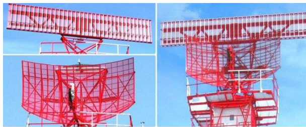
Figure 1. Airport antennae for SSR (left side top) and PSR (left side down). The whole antennae system (right side).
