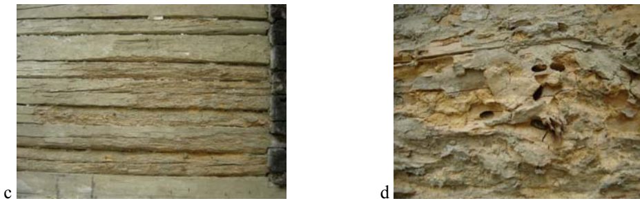
Fig. 11. a, b, c, d – Decay caused to the wood by the combined action of micro-Fungi and the attack of xylophagous insects (original).
